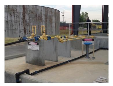
Figure 3-28: NaOCI Unloading Piping
