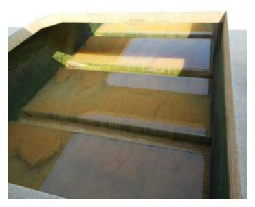
Figure 3-13: Example of Debris in Filter
