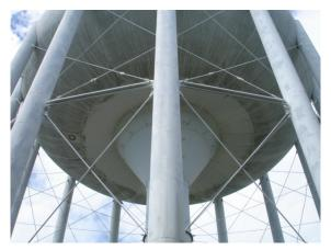
Figure 5-14: Elevated Storage Tank
