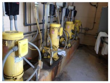
Figure 3-58: Polymer Feed Pumps
