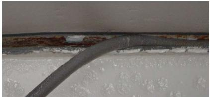
Figure 5-11: Caulking and Backing Rod in GSTs
