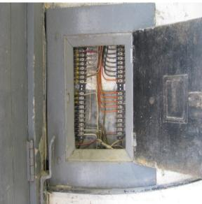
Figure 4-5: Deteriorated Junction Box
