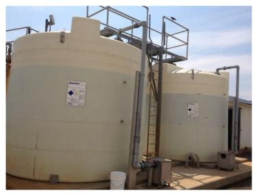
Figure 3-57: Polymer Storage Tanks
