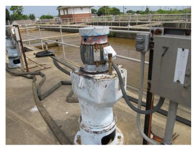
Figure 3-7: L Basin Paddle Driver at Deck Level
