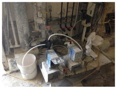
Figure 3-56: Polyphosphate Feed Pumps
