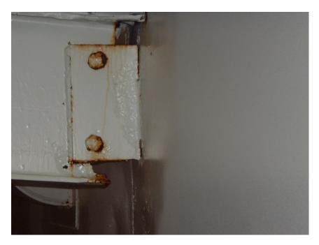
Figure 5-12: Corrosion of GST Roof Beams
