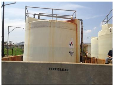
Figure 3-42: Ferric Sulfate Storage
