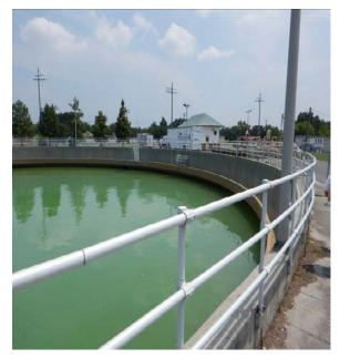
Figure 5-10: Backwash Waste Holding Tank at the Carrollton WTP
