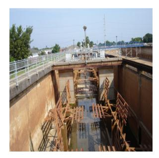
Figure 5-1: Dewatered G3 Basin with Flocculators
