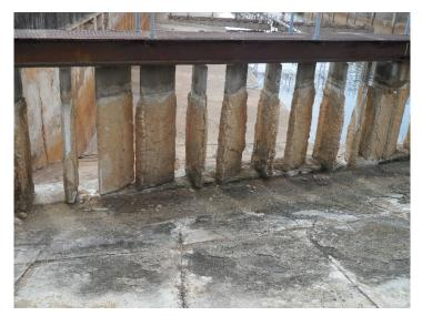
Figure 3-4: G Sedimentation Basin Inlet Butterfly Gates
