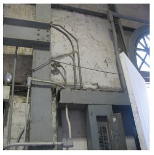
Figure 4-4: Deteriorated Electrical Equipment
