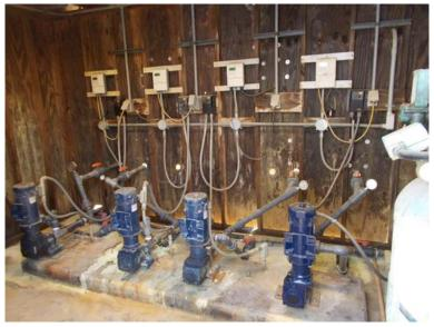
Figure 3-43: Ferric Sulfate Feed Pumps
