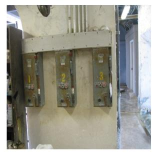
Figure 4-6: Deteriorated Motor Starters
