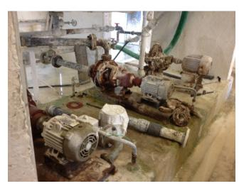
Figure 3-40: Lime Feed Pumps
